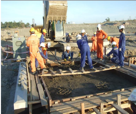
Pouring Concrete for Footing of Pipe Support
