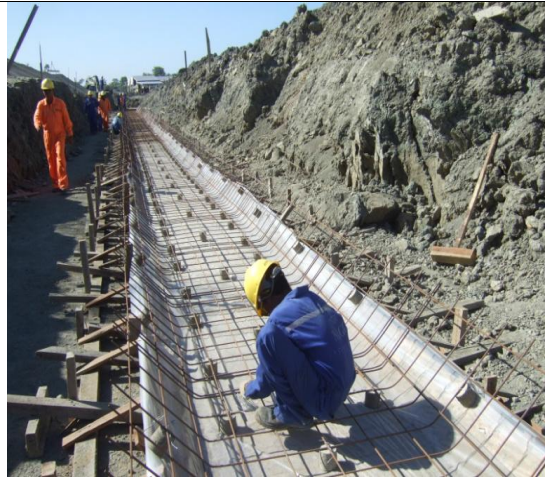
Installation of Wire Mesh for Footing at V Ditch
