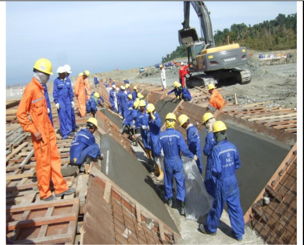
Pouring Concrete for Wall of V-Ditch
