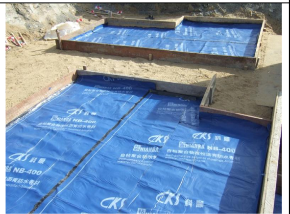
Laying Geo-membrane for Cable Tray Supports
