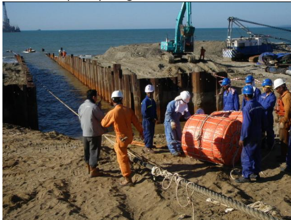
Preparation for Shore Pull Operation
