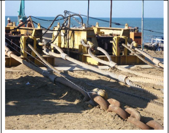
Winch ropes at shore pull operation
