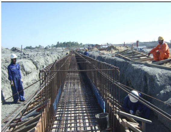
Installation of Rebar for U Ditch
