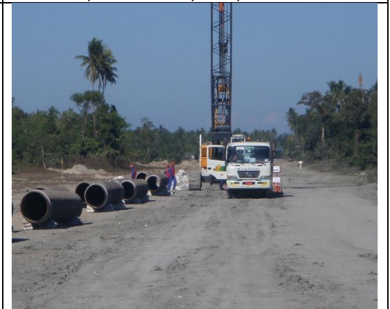
Onshore pipes ready at shore pull area
