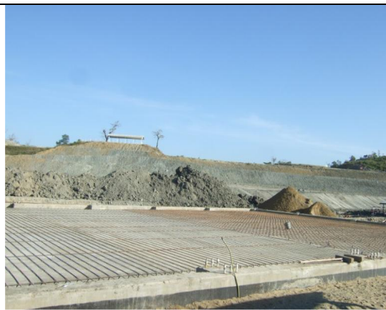
Installation of Rebar for Ground Slab
