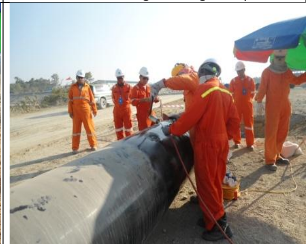
DEP Persons checking Pipeline welding
